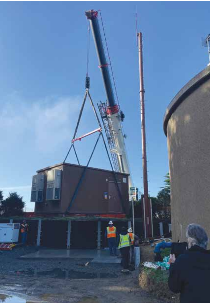
MERA Communications Shelter being placed at the Muir Beach site. Photo by Dave Jeffries
