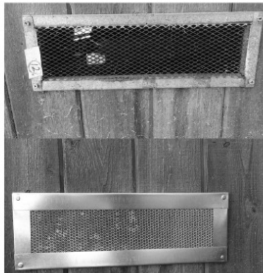
TOP: AN OLD VENT; BOTTOM: VULCAN VENT
