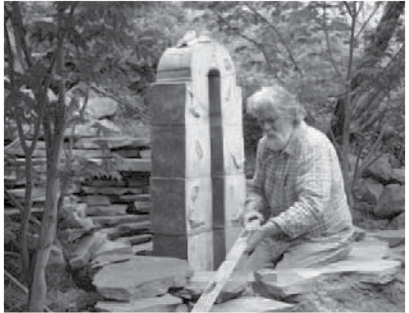
John John installing the fountain at the MBCC. Photo: Laurie Piel
